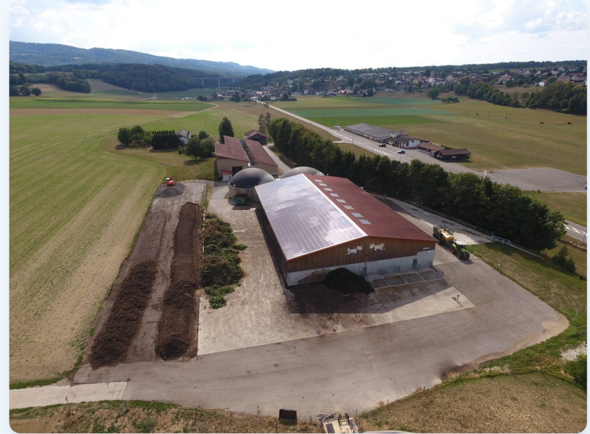
Biogas Plant Site
